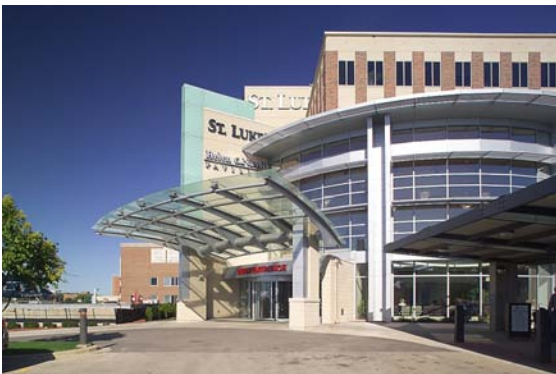
St. Luke's Hospital Iowa Health System
